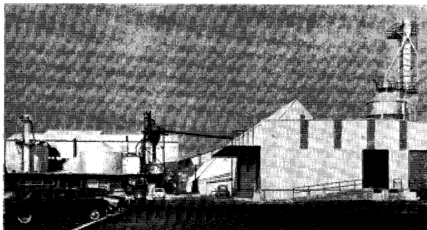
New Calspray plant at Richmond, Calif., was placed on stream Oct. 9. Building at right contains bagging and shipping equipment run by automatic controls
